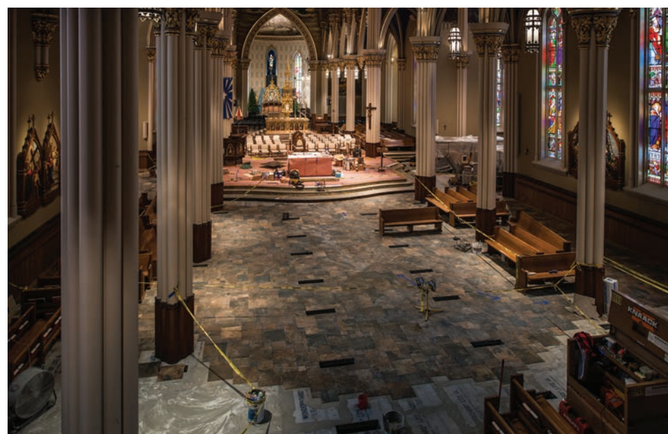
The Basilica of the Sacred Heart recently completed a three-week floor renovation. The carpet was removed and replaced with slate and tile flooring. The Basilica re-opened for Mass on Moreau Day, Jan. 20, 2014.
