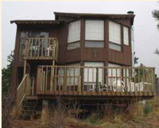
Further up the mountain from Marigreen Pines Novitiate is this house of solitude, built by and routinely used by novices and Novitiate staff
